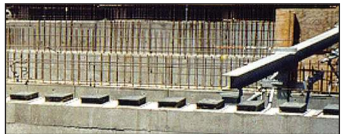
Leveled Isolation Pads Resting on Foundation Wall Prior to Continuing Construction
