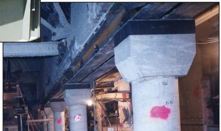
Subway Isolation Pads Under Carnegie Hall
