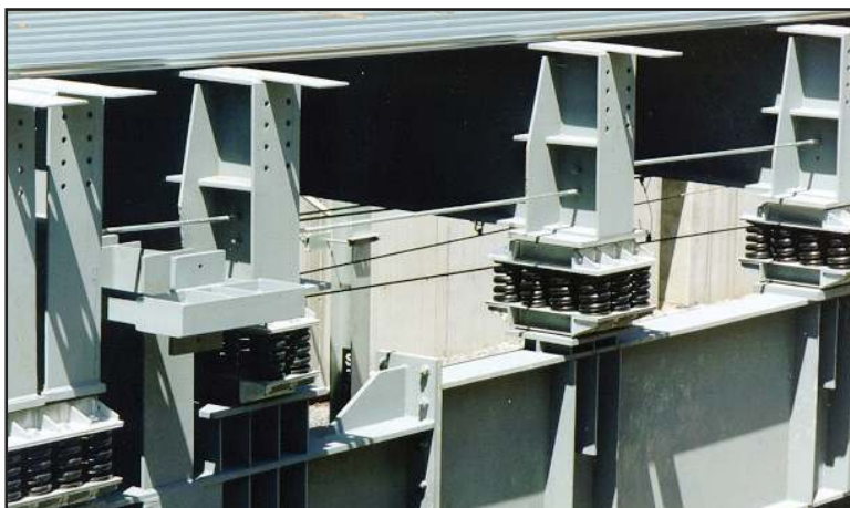
Rubber Isolation Bearing Type BBNR
